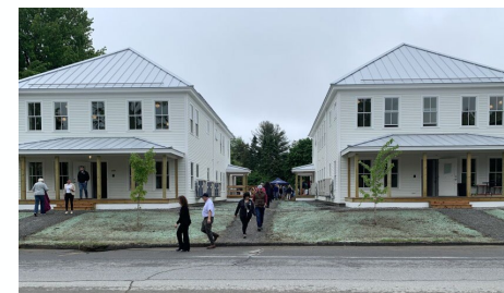
18 Homes Constructed with Modular Units Manufactured by Maine-based KBS Builders in Madison, Maine
