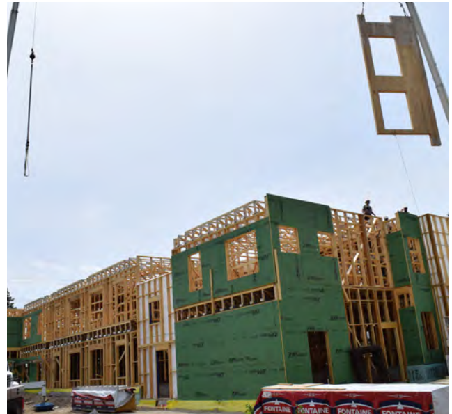
Cross-laminated timber, a value-added and climate-friendly construction material in lieu of steel, is used during construction of a 40-unit apartment building in Portland in summer 2020.
