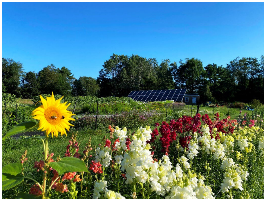
Photo credit: ReVision Energy
