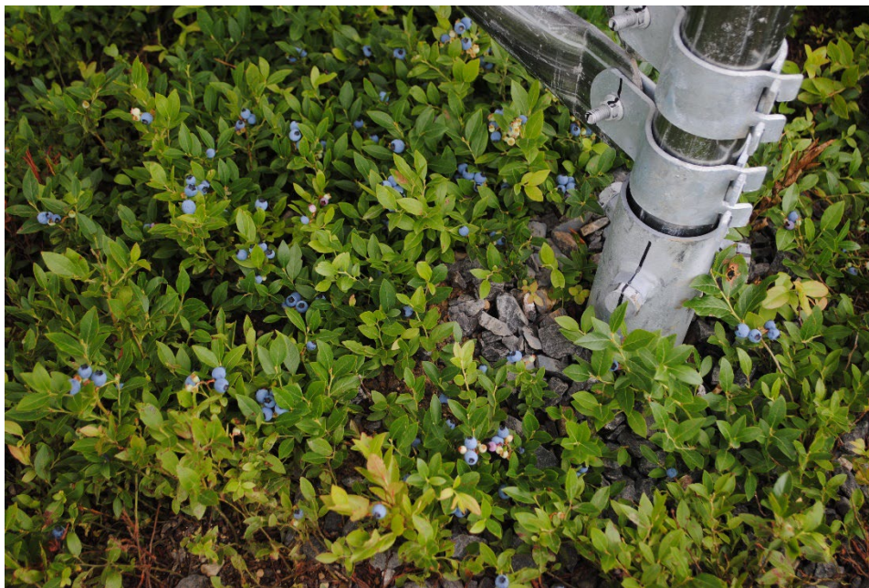
Photo credit: BlueWave Solar
