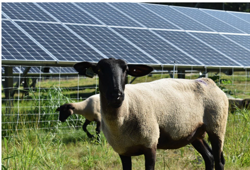
Photo credit: BlueWave Solar
