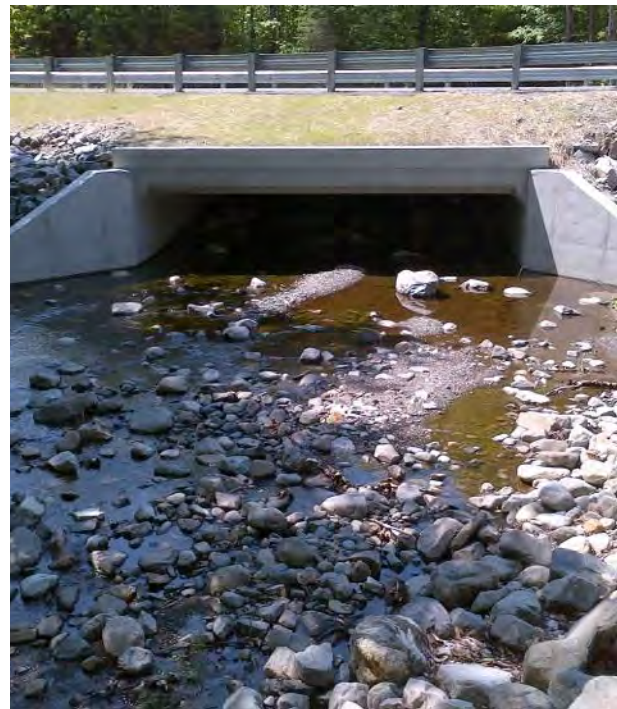
This stream crossing on Bottle Brook in Kingsbury Plantation is an example of a climate-ready infrastructure project that is also geared to improve habitat connectivity.
