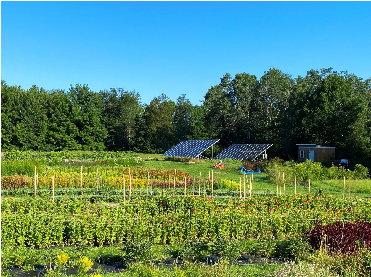
Credit: ReVision Energy
