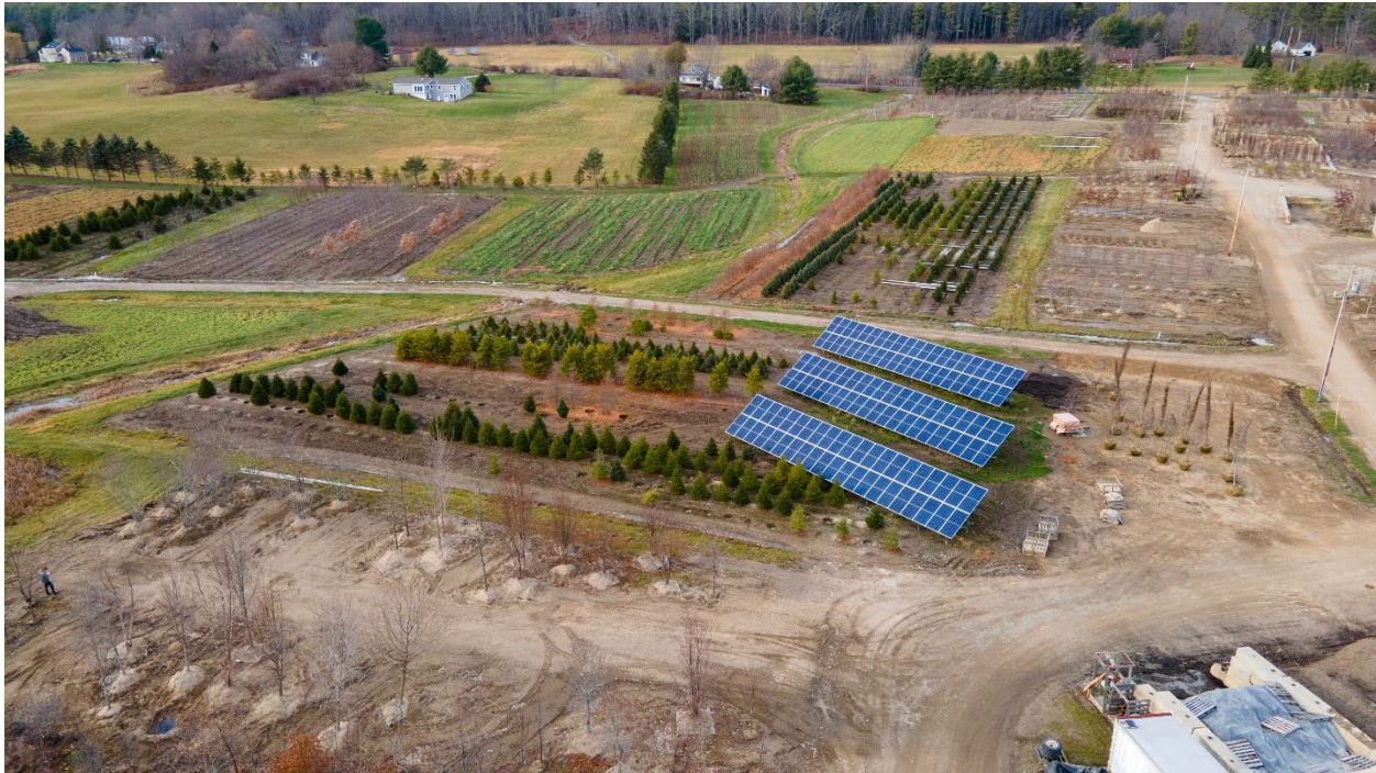
Photo credit: ReVision Energy
