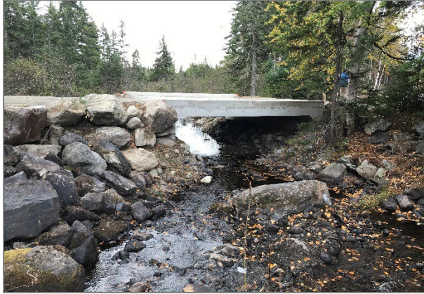
New bridge to enhance fish passage at Cold Stream Forest Unit, BPL Western Region
