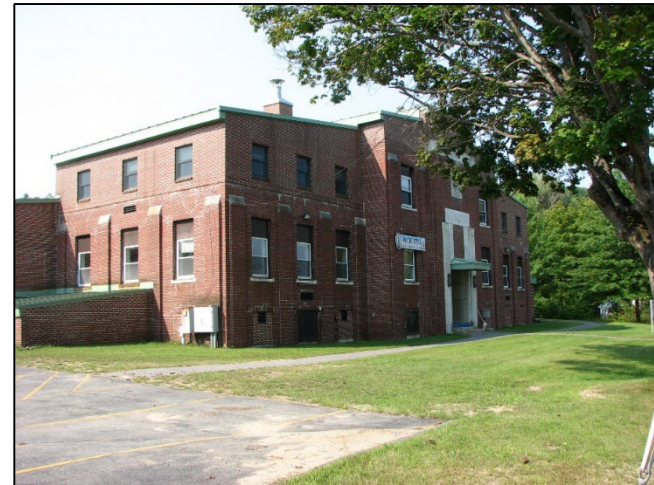
Norway Armory – Future Renovation
