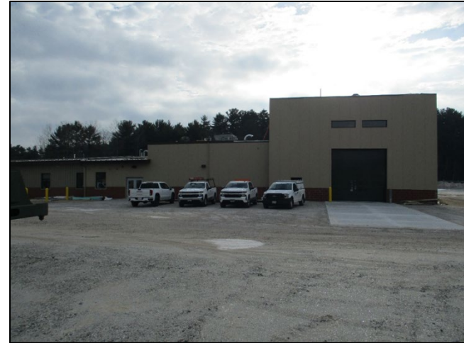
Auburn FMS #2 – Maintenance Bay
